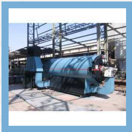
Thermic Heater-Gas Oil Heater
